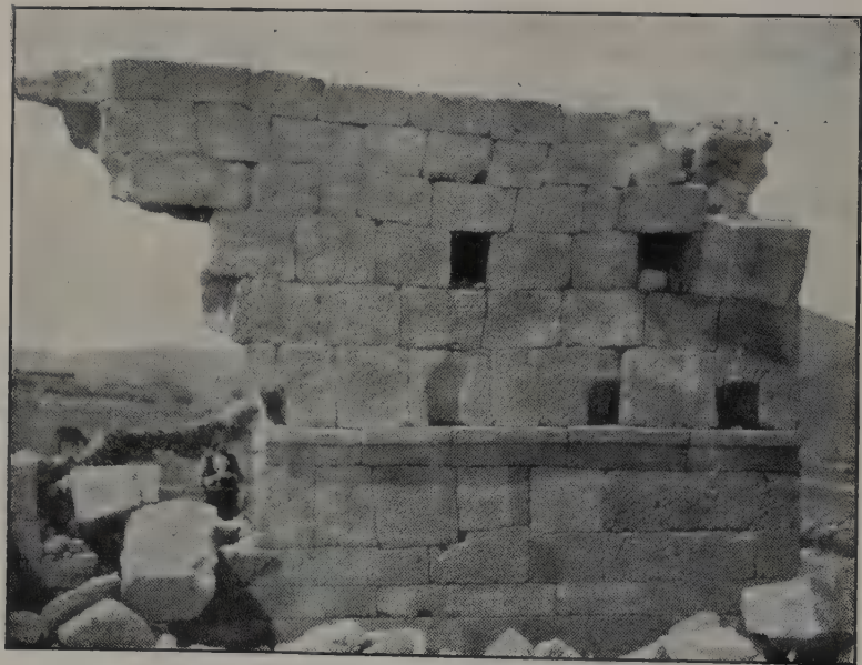
FIG. 76.—No. 11, interior of N. wall of nave.
